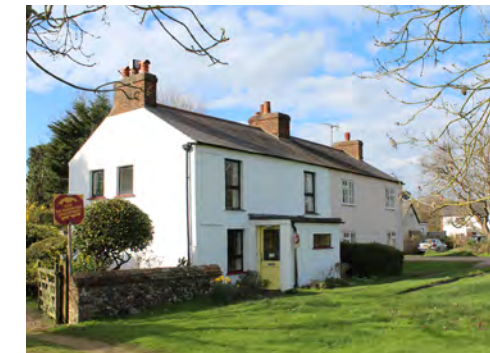
Figure 29 South and Smiths Cottage
